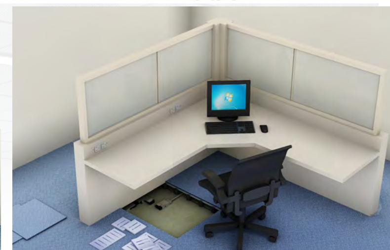
Power to Systems Furniture
